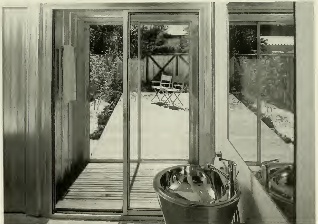
Beginning in the shower, a 4 x 2 pine deck (2 x 4s were turned on edge) continues outside into private garden. Photograph: Neal Bredbeck
